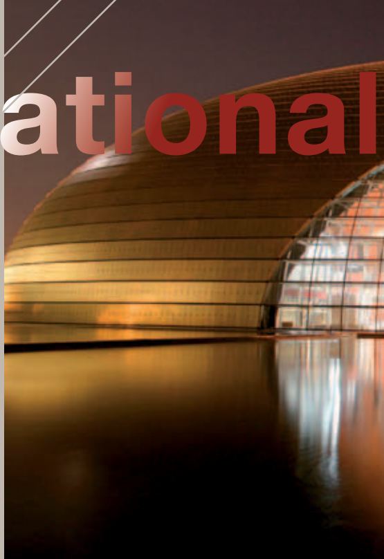
Beijing, National Centre for the Performing Arts, China tour, 2010
